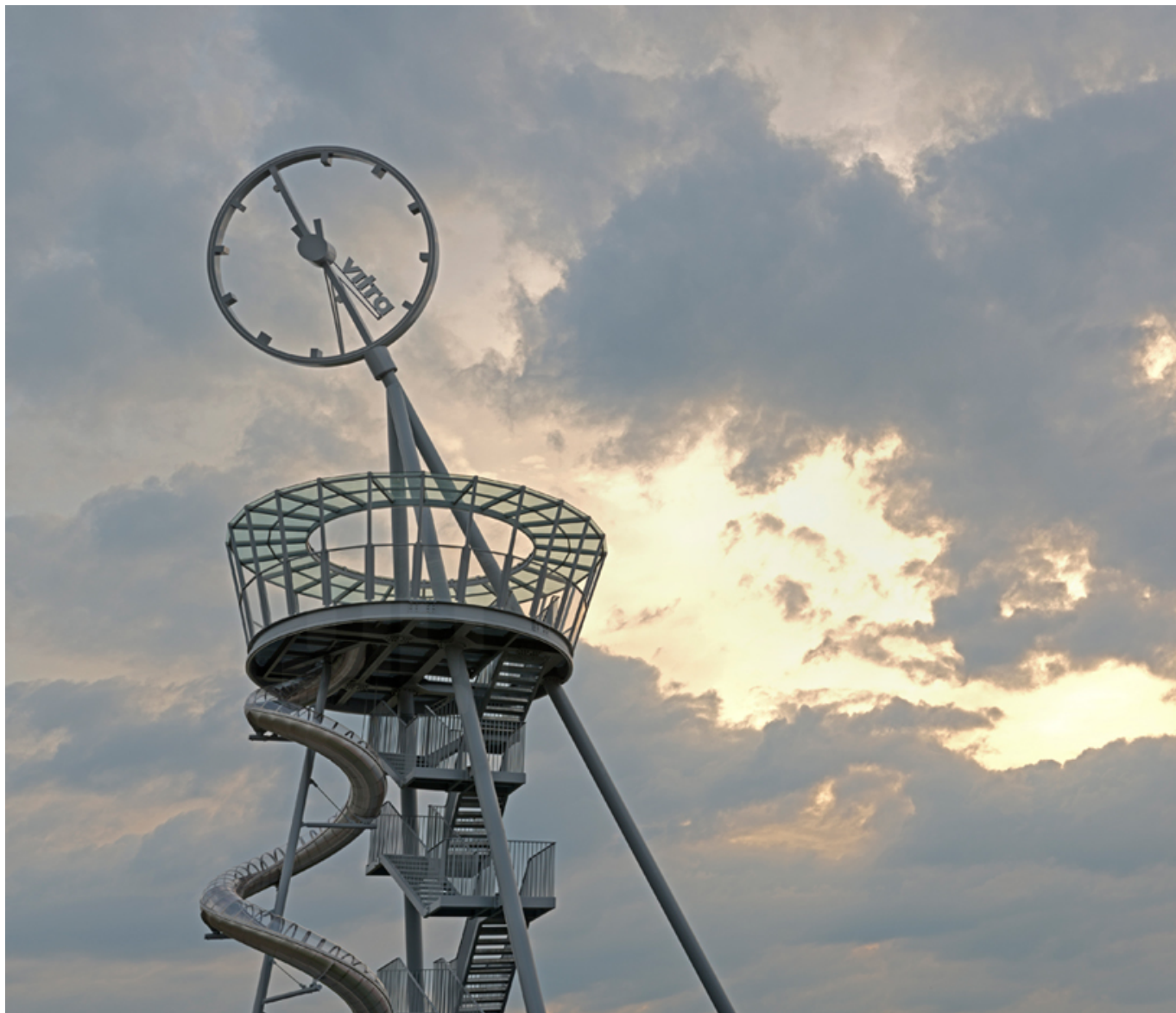
a 6-metre diameter clock sits at the top of the three supporting columns photo by attilio maranzano
